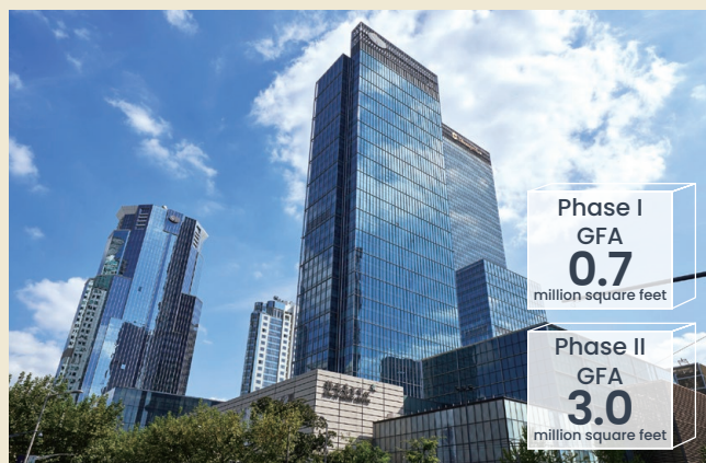
Jing An Kerry Centre, Shanghai
