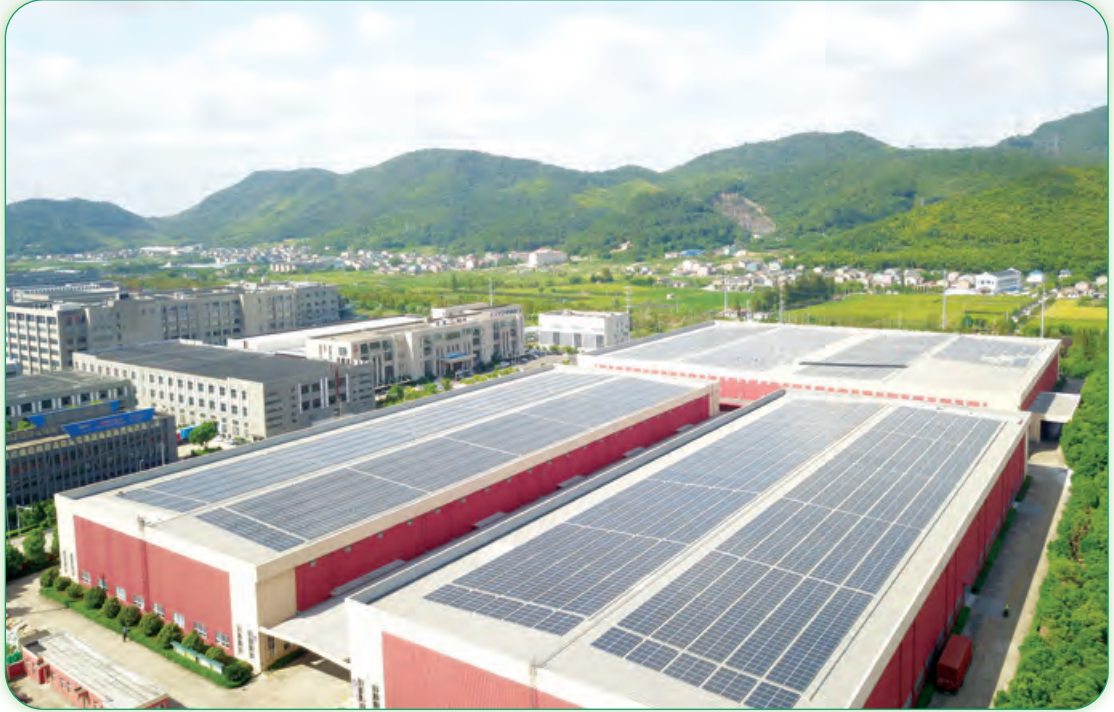
寧波廠區的太陽發電板 PV panels in the Ningbo factory
