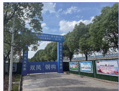
Implement closed construction on site
