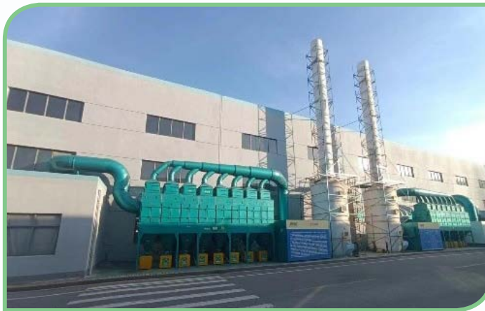
Exhaust gas treatment facility 廢氣處理設施
