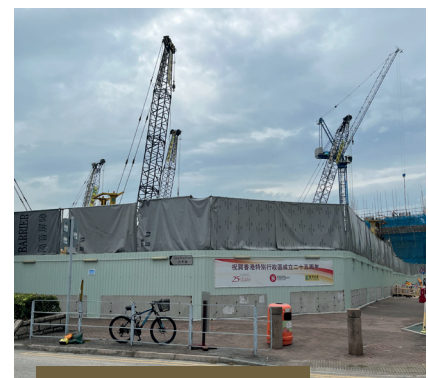
Noise barriers on-site
