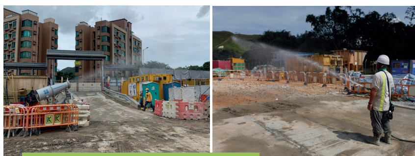
Dust control measures in construction sites
