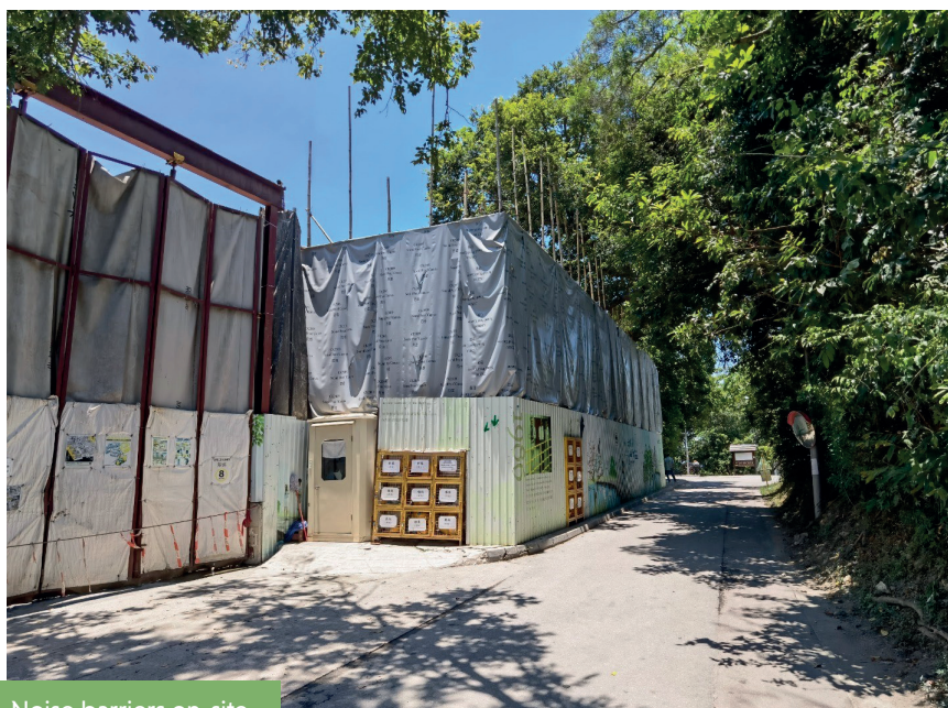
Noise barriers on-site
