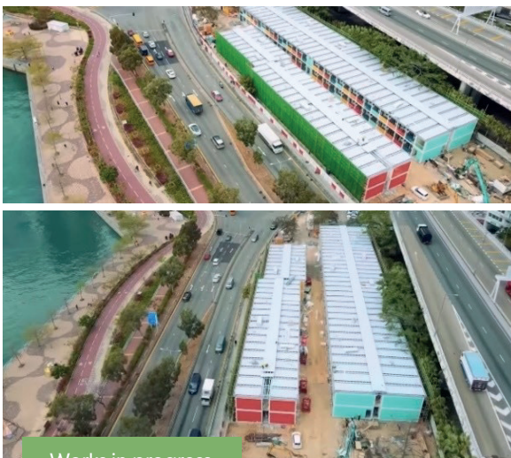
Works in progress
