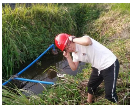
Leakage detection by Lanhe Water Plant
