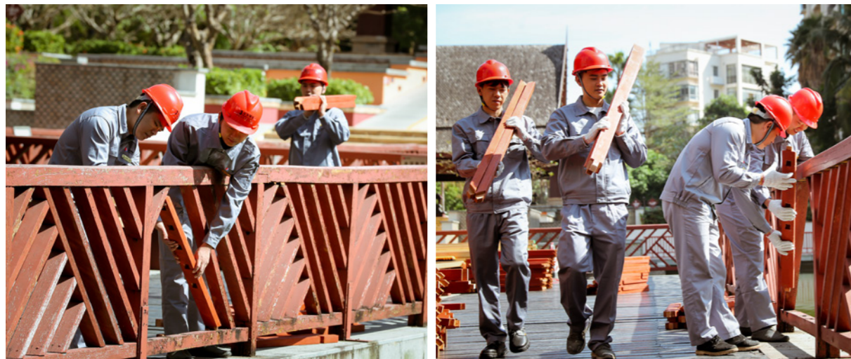
Wooden board of the park's corridor bridge
