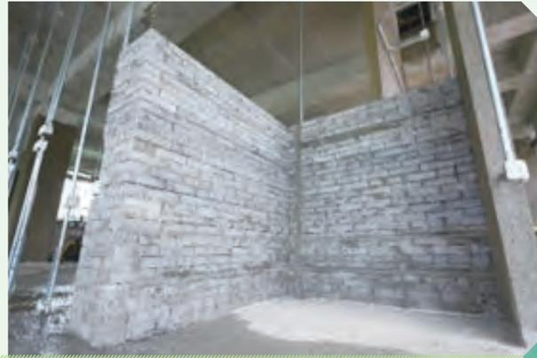
Wall made of the carbon fixation bricks (taken at O-PARK2 site)
