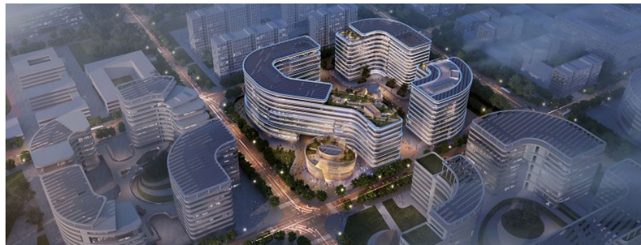
> The integrated energy project in West District I, Fengtai Park of Zhongguancun Science Park
