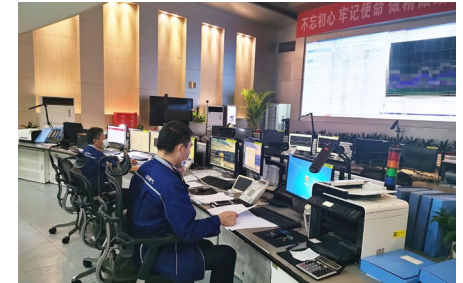
> The SCADA monitoring system in Beijing Gas's operation and dispatch center
