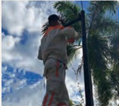
Checks and Maintenance of Street Lights in the Residential Areas
