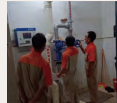
Maintenance of the Drainage Facilities
