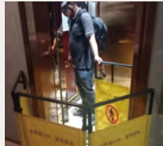
Maintenance of the Lift Operation
