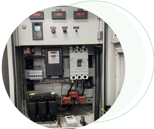
The Yuedong oilfield installed time control switches in variable frequency heating cabinets
