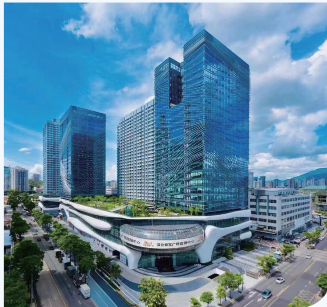
▲ Sponge city sustainable development application of Shum Yip Taifu Square (深業泰富廣場) project
