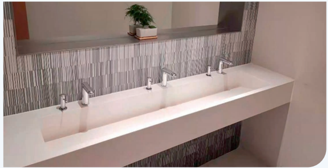
▲ Site picture of installation of water-saving devices
