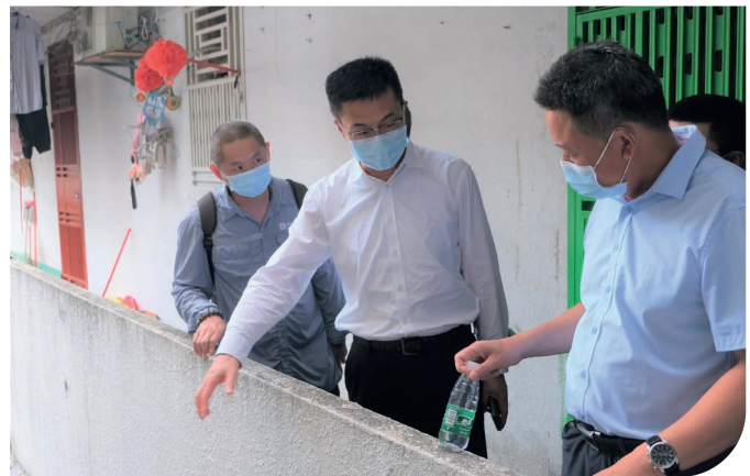
▲ House structure safety inspection
