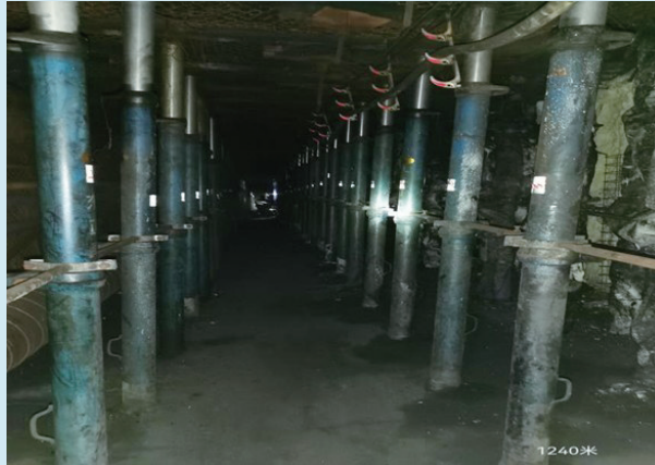
Picture: 110 method – green mining site with no coal pillars along the gob-side entry
