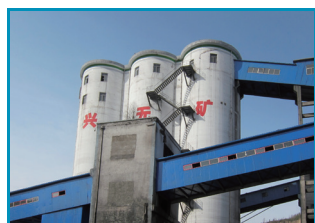
Xingwu Coal Mine 興無煤礦
