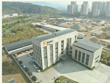
零碳場站現場 The site of zero-carbon station
