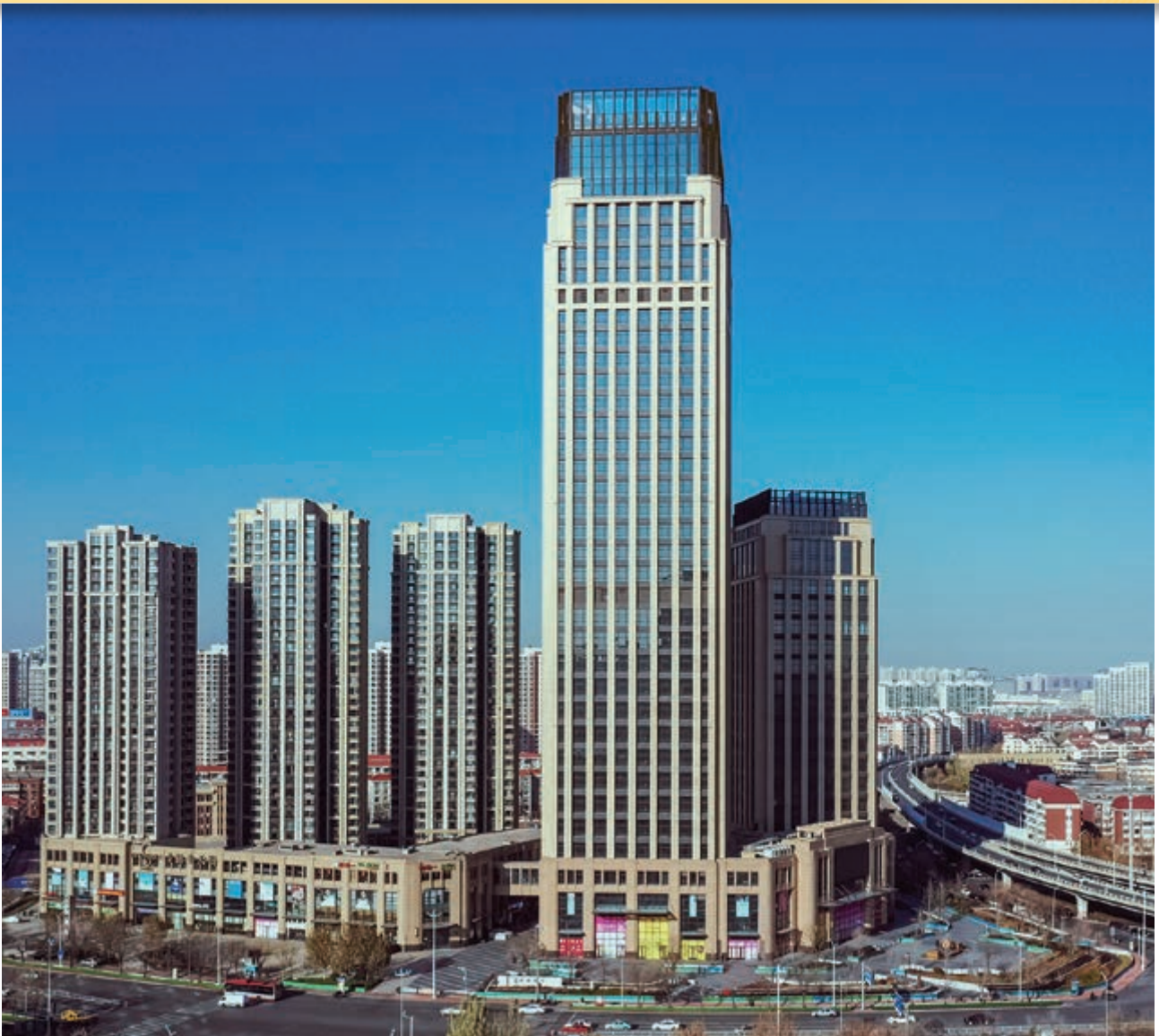
Regal Renaissance, a composite commercial/office/residential development in a prime location of Hedong District, Tianjin
