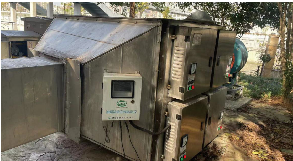
Illustration: Online monitoring device for cooking fume in canteen
