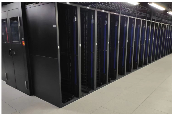
Cold aisle closure system
