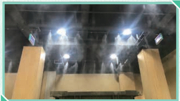
Spray deodorization equipment is installed at the garbage transfer station
