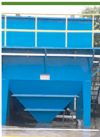
Picture of the sewage sedimentation tank (left) and the sewage facility (right)
