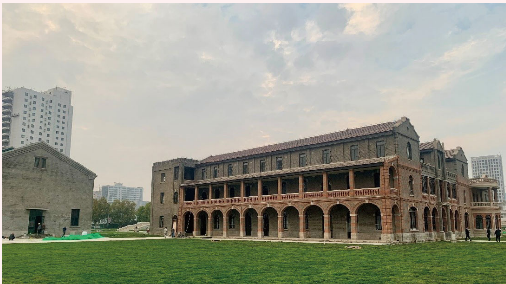
Renovated Shijiazhuang Zhengtai Hotel
