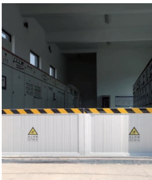
Ossen Innovation Materials Installed Rat Guard on the Door of the Electrical Control Room
