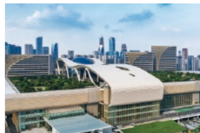
▲ Hangzhou International Expo Center
