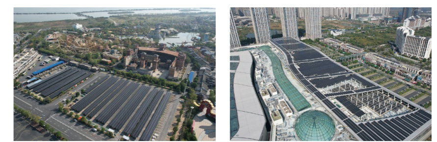
▲ Hefei Sunac Mall PV Power Generation System
