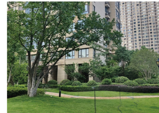
Automatic spraying system
