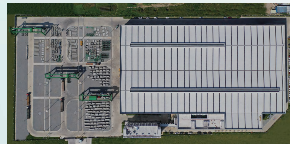
Foshan Photovoltaic Plant
