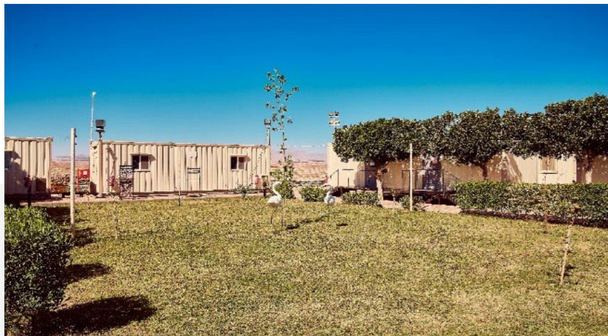
Treated sewage water for green area at KEE
