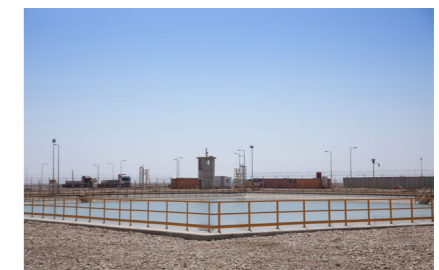
Water treatment plant at KEIL
