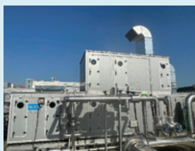
Air-conditioning unit with U-shaped phase-change energy-saving unit
