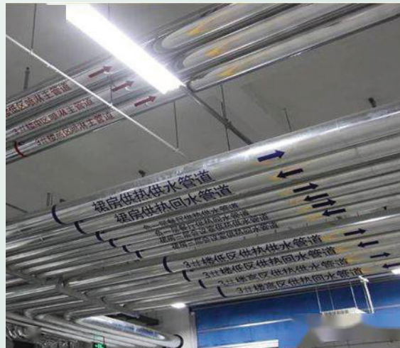
Piping identification illustration
