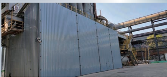
Sound-proof Shield for Coal Injection Heating Furnace of Ironmaking Plant 1 煉鐵一廠噴煤加熱爐隔音棚
