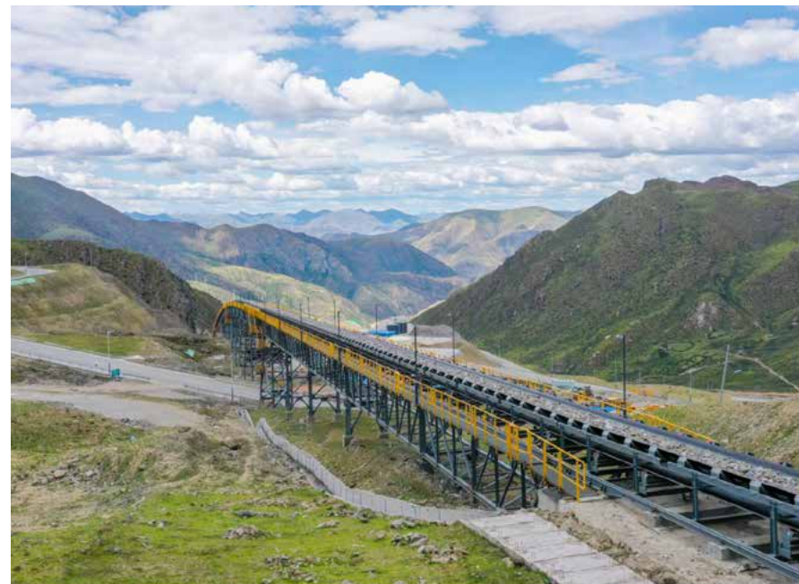
Julong Copper's Long-distance Ore Conveyor Belt Rechargeable on the Downhill Return Movement
