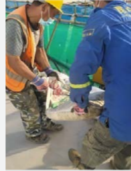
沙袋防汛 Using Sandbags for Flood Protection
