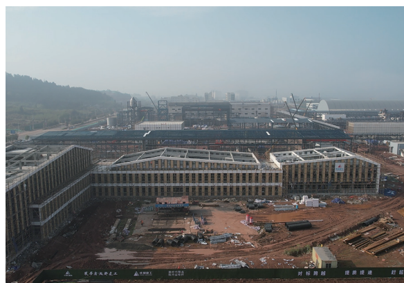
The construction site of Anju project
