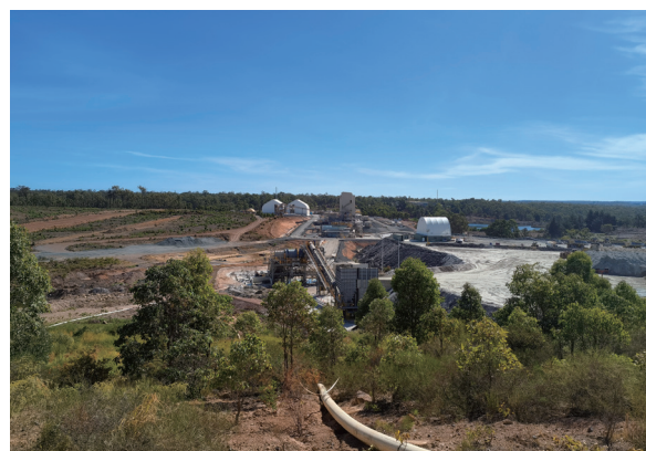
Greenbushes Tailings Treatment Plant
