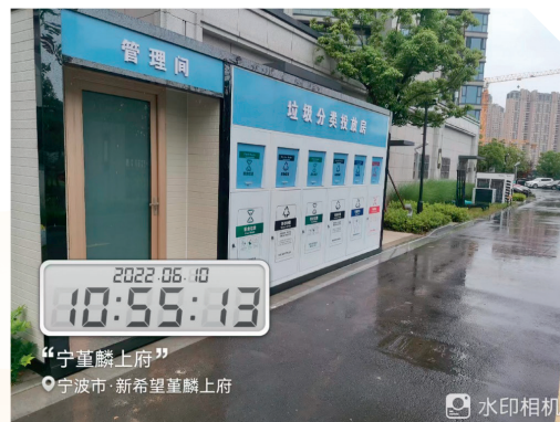
Standardisation of domestic waste sorting in Ningbo Jinlin Mansion (寧波董麟上府), with a fully enclosed garbage chamber to give owners a good sense of quality
