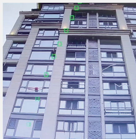
Ouwang Mansion – cameras for monitoring things thrown off the buildings
