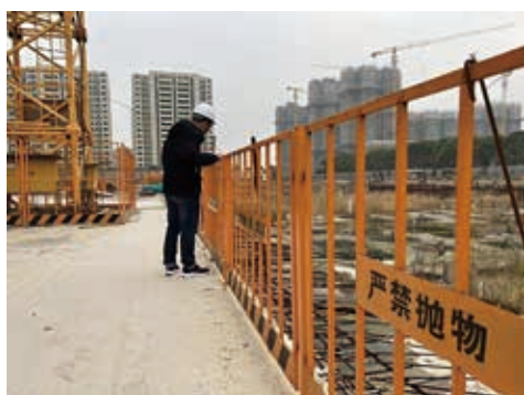
Inspection workers are examining whether the edge and opening protection is sufficient to ensure workers' safety
