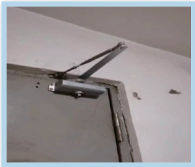
Replacement of the damaged door closer
