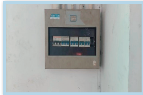
Replacement of the damaged power distribution box cover
