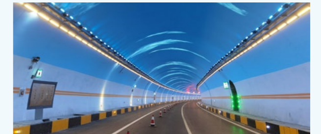
二航局、一局集团承建的延庆至崇礼高速公路河北段 Hebei Section of Yanqing-Chongli Expressway undertaken by CCCC Second Harbor Engineering Company Ltd. and CCCC First Highway Engineering Group Co., Ltd.
