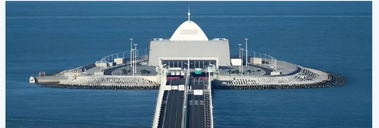
中国交建承建的港珠澳大桥主体工程岛隧工程 Island tunnel engineering, the main works of Hong Kong-Zhuhai-Macao Bridge, undertaken by China Communications Construction
