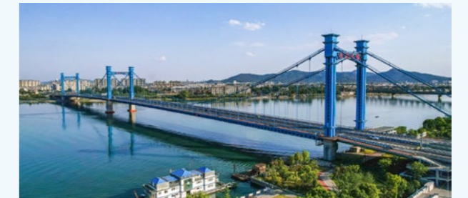
二航局承建的襄阳庞公(凤雏)大桥 Xiangyang Pangong (Fengchu) Bridge undertaken by CCCC Second Harbor Engineering Company Ltd.
