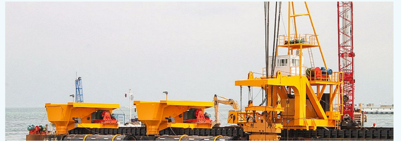
一航局：深水基床夯实系统 CCCC First Harbor Engineering Company Ltd.: Deep-water Foundation Bed Tamping System
