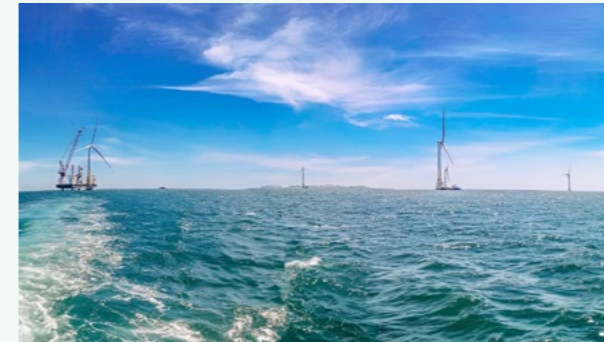
国内首个成规模单机容量 5 兆瓦直驱型风机的海上风电场——中闽福建平海湾海上风电场 First large-scale offshore wind farm in China with a single unit capacity of 5 MW with direct-drive fan - Zhongmin Fujian Pinghai Bay Offshore Wind Farm
