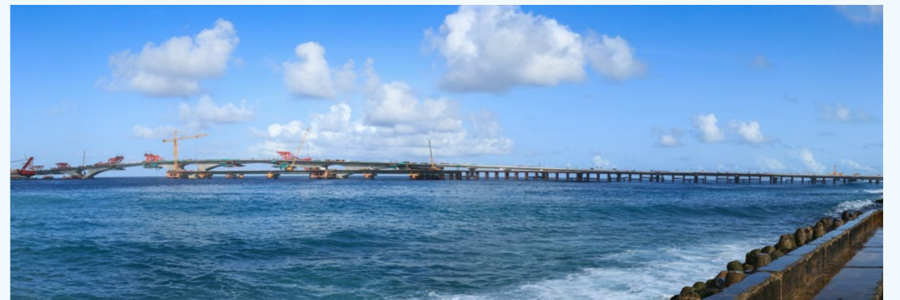
二航局：钢混叠合的混合梁桥施工方法（援马尔代夫中马友谊大桥） CCCC Second Harbor Engineering Company Ltd.: Mixed Beam-bridge Construction Method with Steel and Concrete Superimposed China-Maldives Friendship Bridge for the Support Project of Maldives
