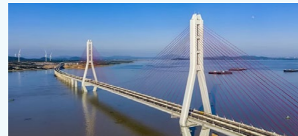
中国路桥承建的都昌至九江高速公路鄱阳湖二桥 The Second Poyang Lake Bridge of Duchang-Jiujiang Expressway undertaken by China Road & Bridge Corporation
