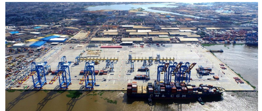
中国港湾承建、一航局施工的科特迪瓦阿比让港第二集装箱码头堆场投入运营 The yard of the second container terminal in Abidjan Port, Côte d'Ivoire, which was built by China Harbour Engineering Company Ltd. and constructed by CCCC First Harbor Engineering, was put into operation
