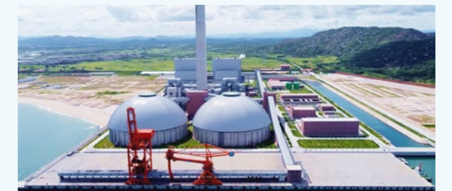
四航局承建的广东陆丰甲湖湾电厂新建工程配套码头工程 Auxiliary Wharf Works of New Guangdong Lufeng Jiahuan Power Plant undertaken by CCCC Fourth Harbor Engineering Co., Ltd.
