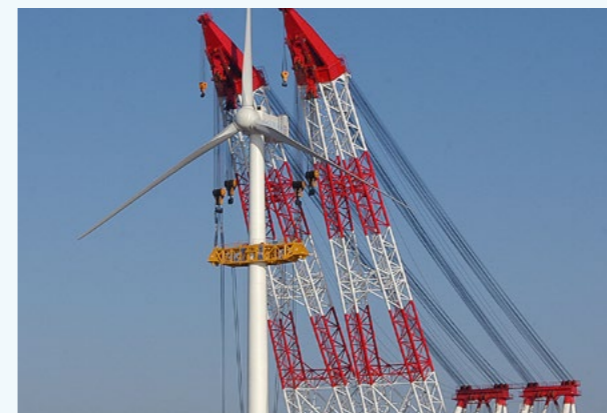
三航局：一种导管架基础精定位及临时锁定系统 CCCC Third Harbor Engineering Company Ltd.: A System of Precise Positioning and Temporary Locking of Jacket Foundation
