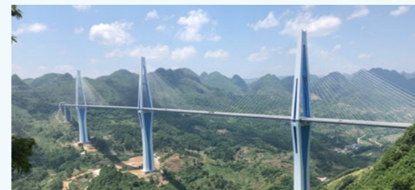
二公局承建的平塘特大桥 Pingtang Bridge undertaken by CCCC Second Highway Engineering Co., Ltd.
