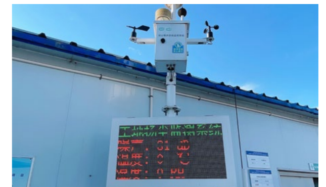
工地扬尘监控系统 Dust monitoring system on construction site
