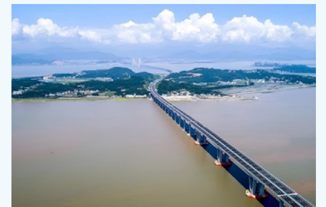
一公局集团：一种变截面节段梁短线预制拼装方法（乐清湾大桥） CCCC First Highway Engineering Group: A Short-line Prefabricated Assembly Method of Variable Cross-section Segment Beams (Yueqing Bay Bridge)
