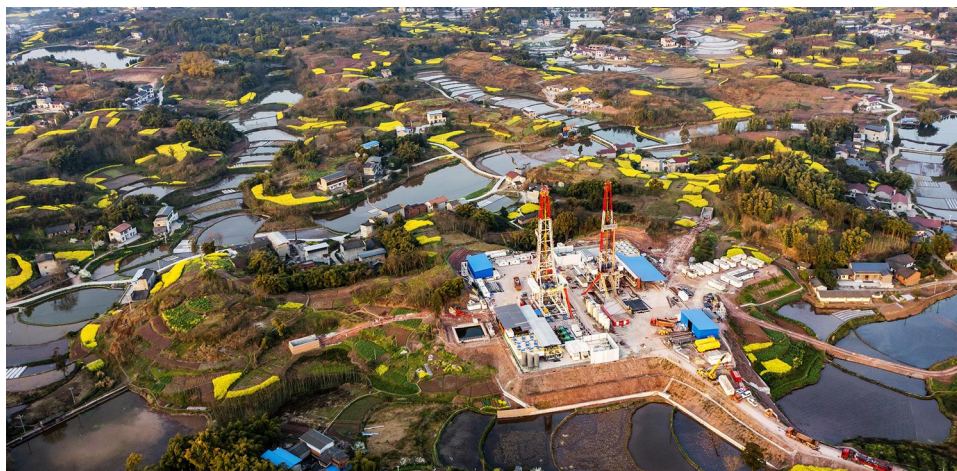
Anton southwest drilling site viewed from Platform 205H1
