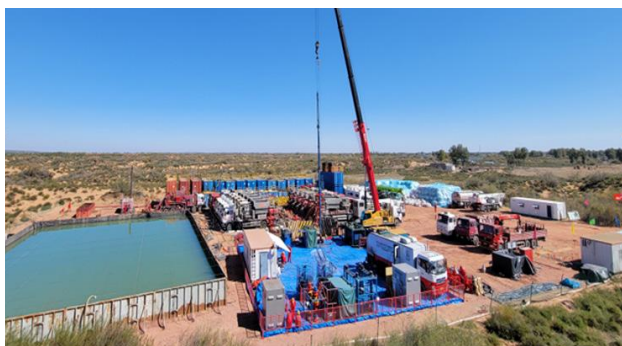
DX-PXX platform fracturing construction site
