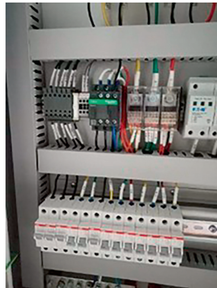
Lighting switch retrofit
