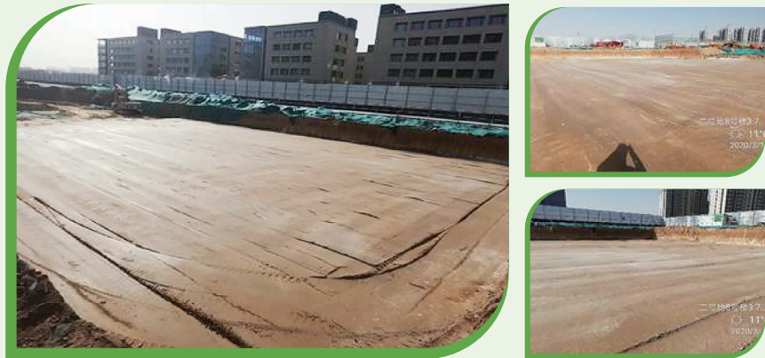
Lime soil backfill in Changsha
