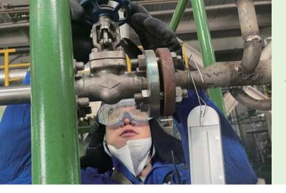
Adjusting refill valve of ammonia pump tank
