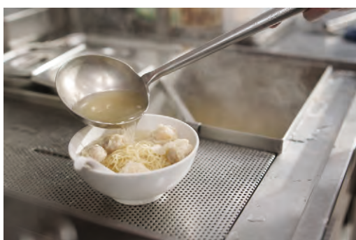
Upgrade of bain-marie heating coils to improve energy efficiency 更換熱湯池的加熱線圈以提高能源效益
