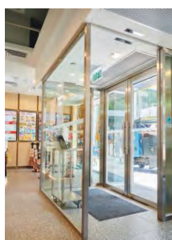
"Air Lobby" at outlets to optimise the efficiency of air conditioning 分店採用「空調大堂」以優化空調效率
