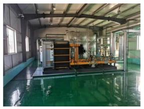
Heat exchange stations are constructed for heat transmission from primary distribution networks to secondary distribution networks. These stations are equipped with heat exchangers, circulation pumps, make-up water pumps, valves, instruments, meters, strainers, water tanks, electric power distribution cabinets, control cabinets and water treatment equipment.
