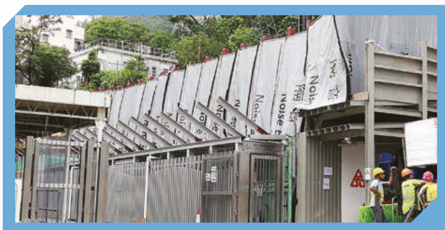
▶ Noise barriers hang on the hoarding 於圍板繫上隔音屏障
