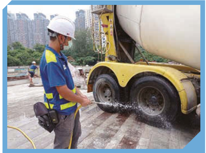
Designated wheel washing area at site 於地盤設立輪胎清洗位置
