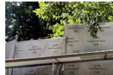
Noise barrier is installed along the site boundaries
