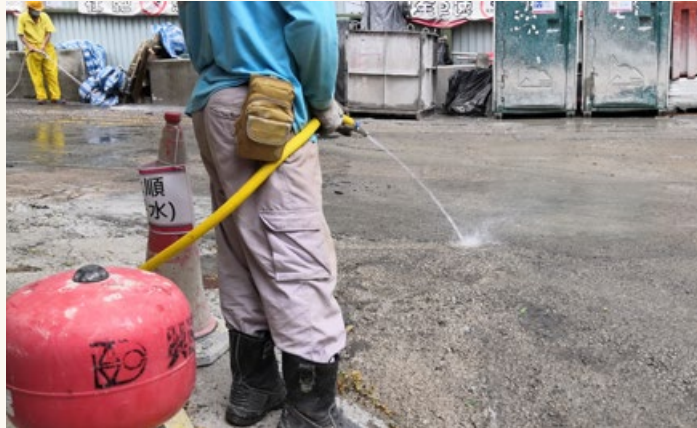
Automatic water pump for cleaning the wheels of vehicles with the use of recycled water
