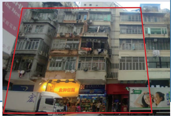
Castle Peak Road re-development project site at Sham Shui Po 深水埗青山道重建項目地盤
