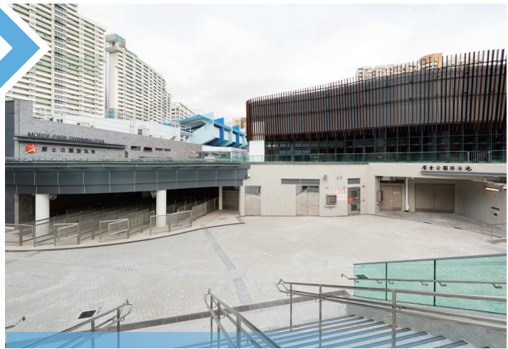
Electrical works for the construction of Siu Ho Wan Water Treatment Works Extension and Siu Ho Wan Raw Water Booster Pumping Station
