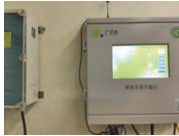
Sewage pollutant monitoring devices installed at the Zhongshan factory
