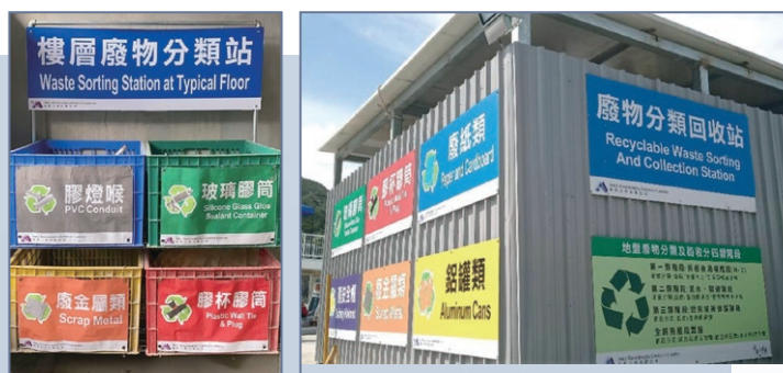
Set up waste sorting stations to improve cleanliness and tidiness of sites 設立廢物分類站，以改善地盤的整潔度
