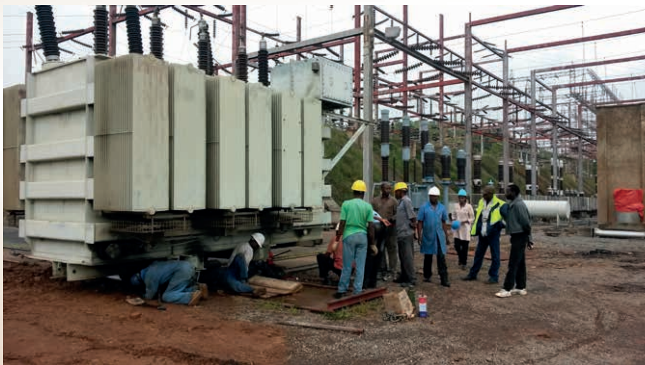
Huachin Leach assisted GCM to make urgent repair on the transformer
