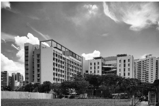
Nursing Home at the North of Singapore
