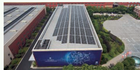
Solar panels installed at a partner factory
